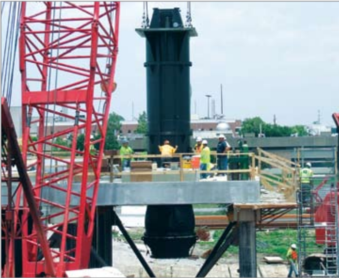
One of eight Patterson pumps being installed at the London Avenue Canal pumping station.
